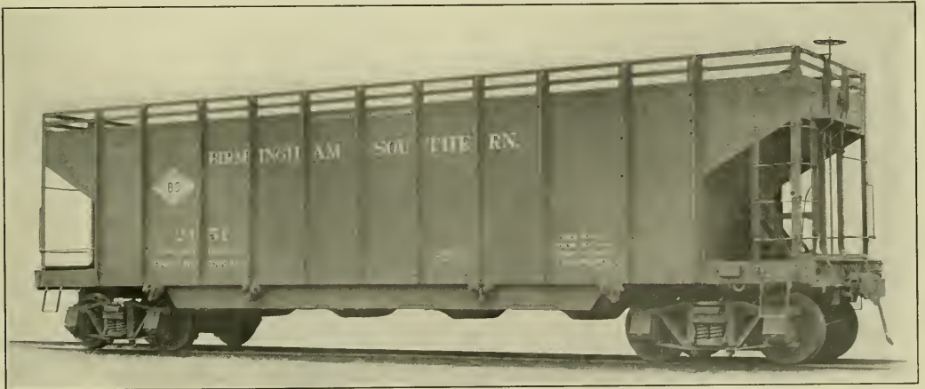
Seventy-Ton Capacity Car with Four Hoppers.
